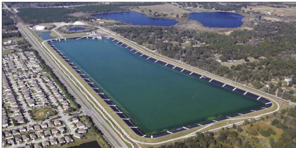
Figure 2. Boyette Road Reclaimed Water Reservoir.
