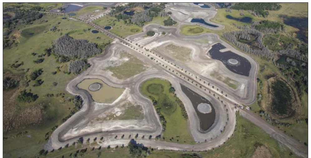
Figure 4. The 4G Wetlands project's constructed wetland cells under construction.
